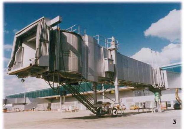
Installation at Stansted Airport 5 x 315 KVA, 400 Hz Bridge Gate Cubicle with Cable Hoist
